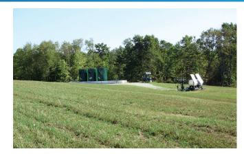
Once drilling is completed, the well pad is reclaimed and revegetated as shown above. Equipment about the size of a two-car garage remains, including the wellhead, water storage tanks and a monitoring system to ensure the long-term operation and safety of the well.
